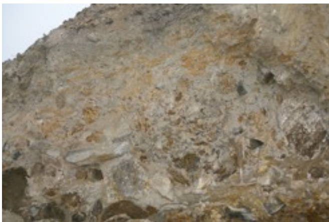
Figure 2: Exposure of what appears to be lower till in the wall of the retention basin. Note the fine-grained, deformed matrix and tightly packed cobbles and boulders. Some of the boulders may look competent, but some could be readily crumbled by scraping with the hammer shown for scale (Harold Moritz photo).
